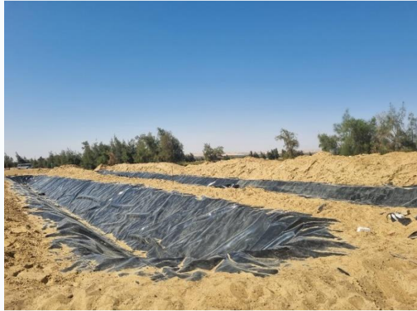
Figure 12. Finishing the construction of the two underground (down-stream) tanks and the poly ethylene lining materials of the two cells and four tanks
