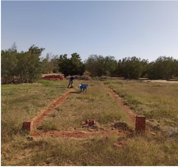
Figure 8. Marking the site of the CWT pilot in Sekem El-Wahat farm, Egypt
