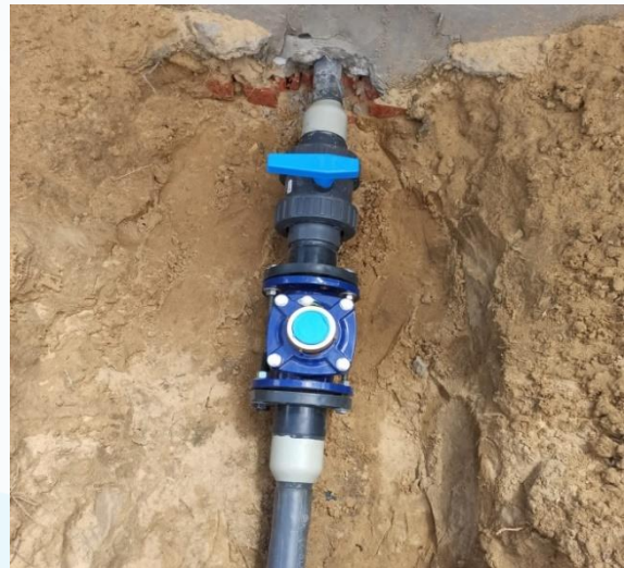
Figure 14. Installing the flow meters and valve at each water tanks (four tanks)
