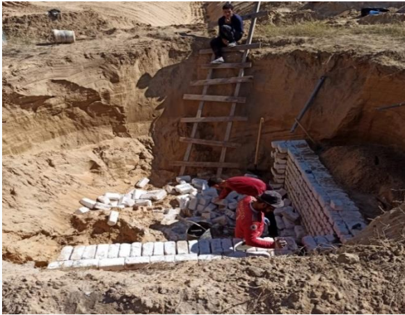
Figure 12. Finishing the construction of the two underground (down-stream) tanks and the poly ethylene lining materials of the two cells and four tanks
